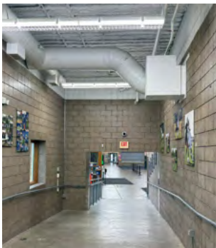
Hallway to dome
