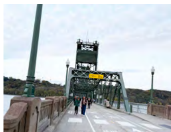
Lift Bridge entrance
