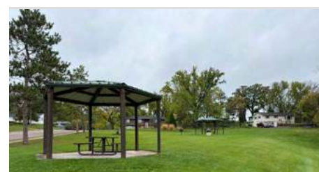
Northland Park small picnic shelter
