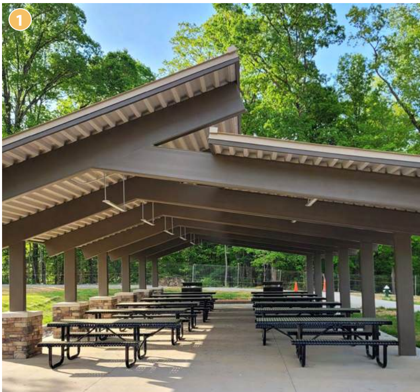
Large picnic shelter
