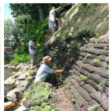
Bio-bag Erosion Control/ Slope Restoration
