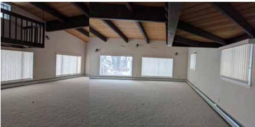
Existing pool room (pool is covered). January 27, 2020.
