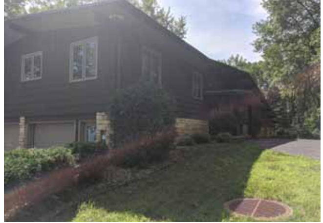
Tuck-under garage and entry (northwest side of building). July 15, 2020.
