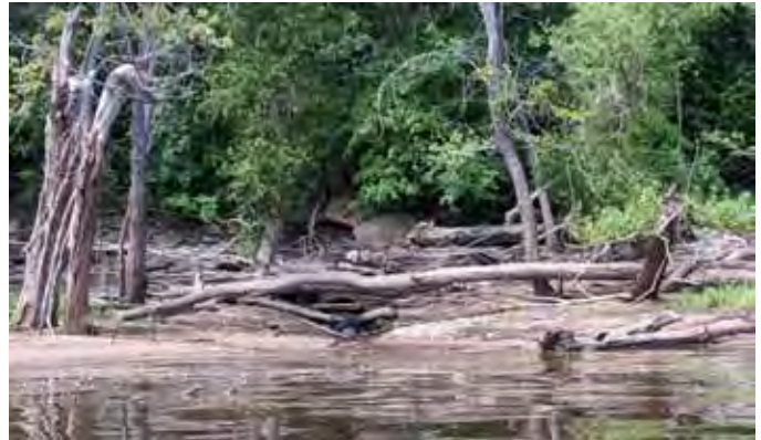
Pond outlet structure under downed trees (view from water looking west). July 15, 2020.
