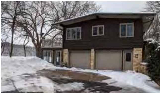
Existing tuck-under garage (north-facing facade). January 27, 2020
