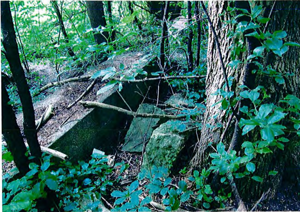
Photo 1: Retaining wall observed parallel to Highway 95 on southern edge of Property
