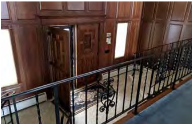
Existing split-level entrance. January 27, 2020.
