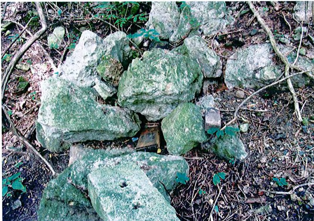
Photo 2: Concrete and brick debris observed throughout the Property
