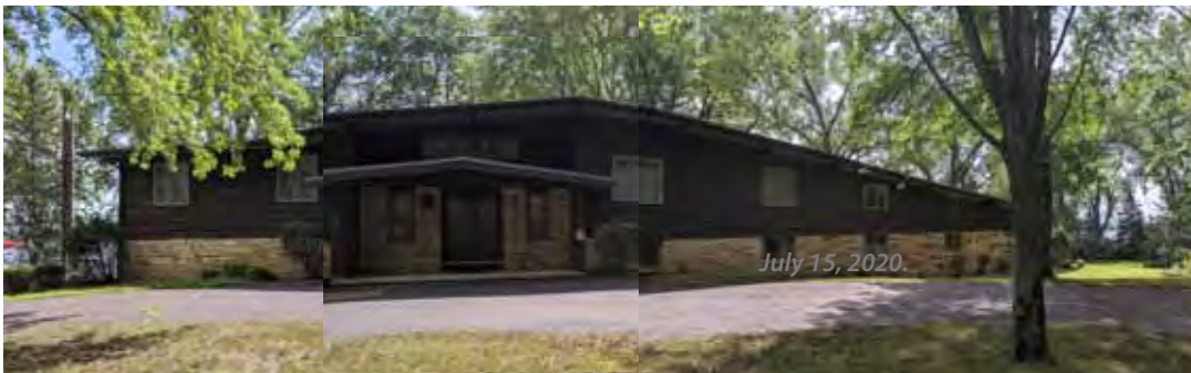
West-facing facade of house. July 15, 2020.
