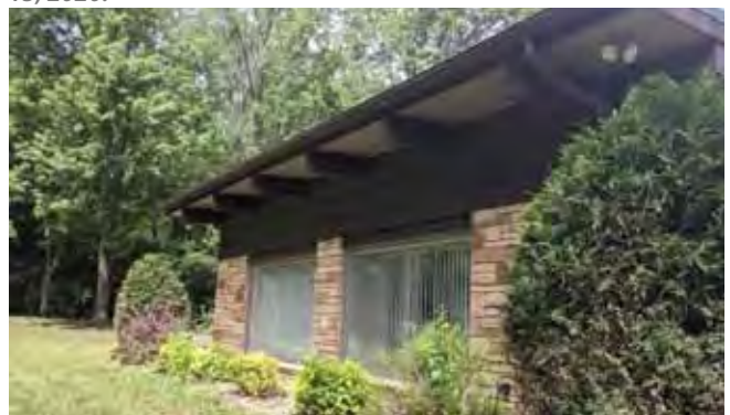
South-facing facade (windows to pool room). July 15, 2020.
