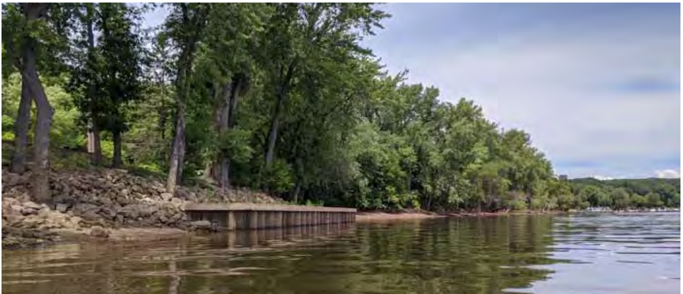
View of steel sheetwalls and beach in background (view from water, looking northwest). July 15, 2020.
