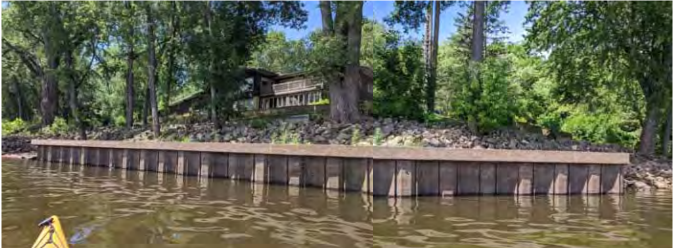
On the river, looking west toward the Aiple residence and over the existing steel sheetwalls that were used for boat docking. July 15, 2020.
