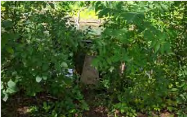
Pond outlet structure with pond in background (looking west from berm footpath). July 15, 2020.
