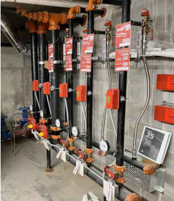
Sprinkler system layout in a commercial building.
